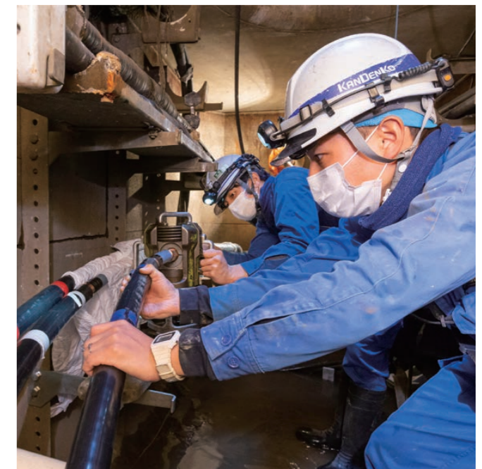
Cable connection work for underground distribution lines facilities (Tokyo)
