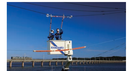
Overhead power distribution line work using the indirect hot-line method
