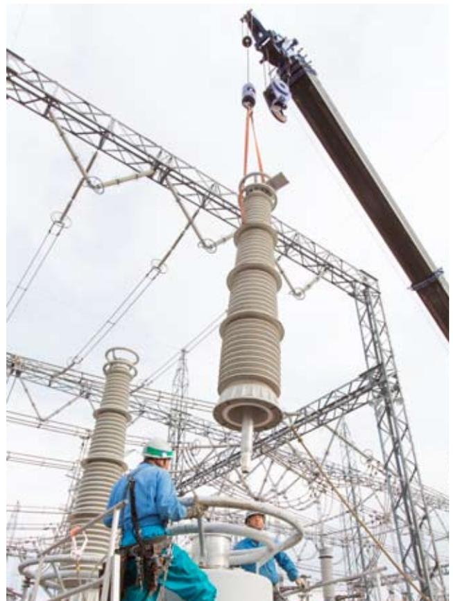
Removing a gas circuit breaker from a transformer at a substation
