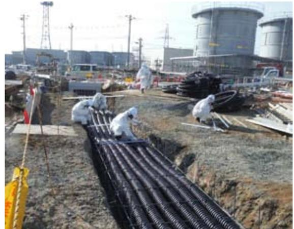
Laying electric power cables in a frozen soil impermeable wall
