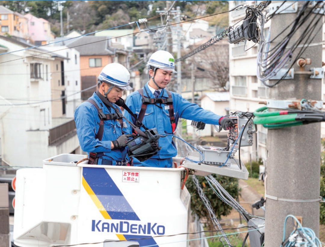
CATV cable installation work (Kanagawa Prefecture)
