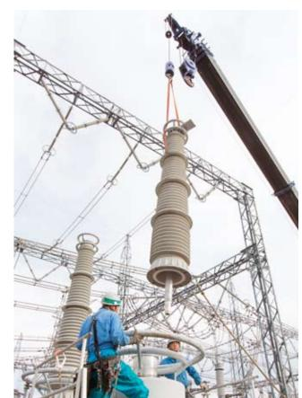
Removing a gas circuit breaker from a transformer at a substation
