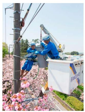
Using an elevating work platform to install a new transformer on a power pole
