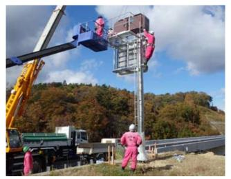
Installing a variable-message sign on a roadway
