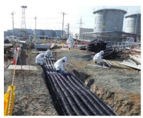
Laying electric power cables in a frozen soil impermeable wall
