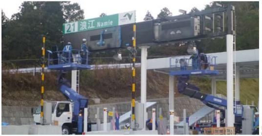
Installing an ETC card-reader gate at the Namie Interchange
