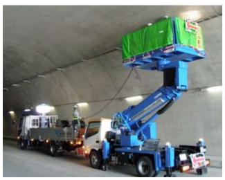
Installing light fixtures in a roadway tunnel
