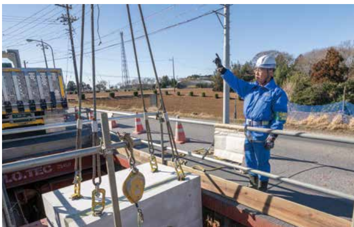
Electrical manhole installation (Ibaraki Prefecture)
