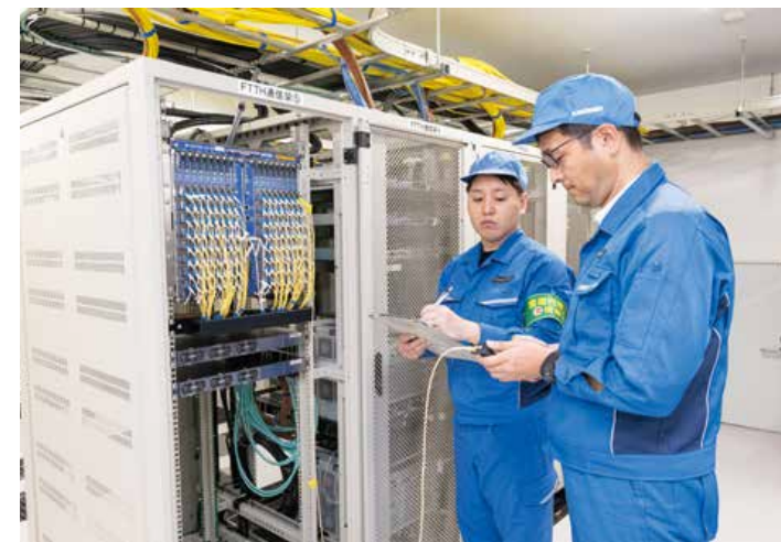
CATV FTTH construction work (Kanagawa Prefecture)
