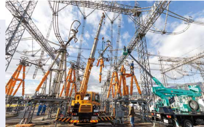
Replacement of switches in substations (Shizuoka prefecture)
