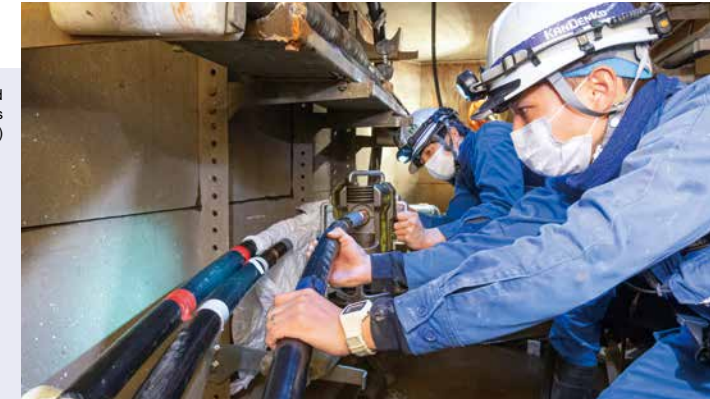
Cable connection work for underground distribution lines facilities (Tokyo)
