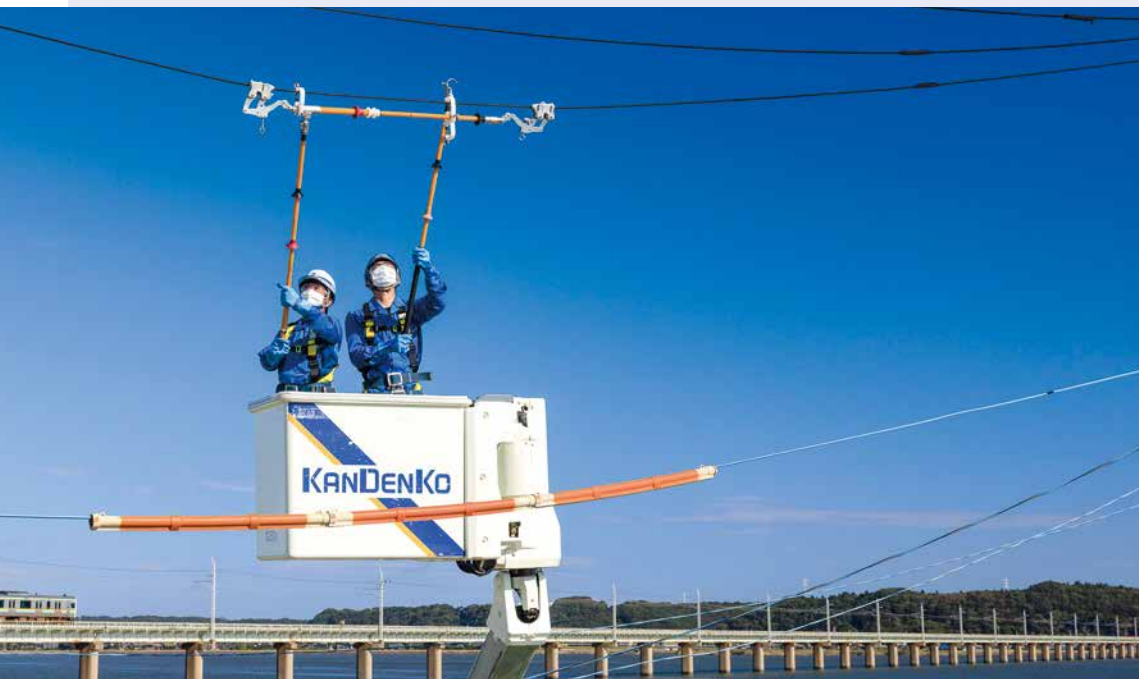
Overhead power distribution line work using the indirect hot-line method (Ibaraki Prefecture)
