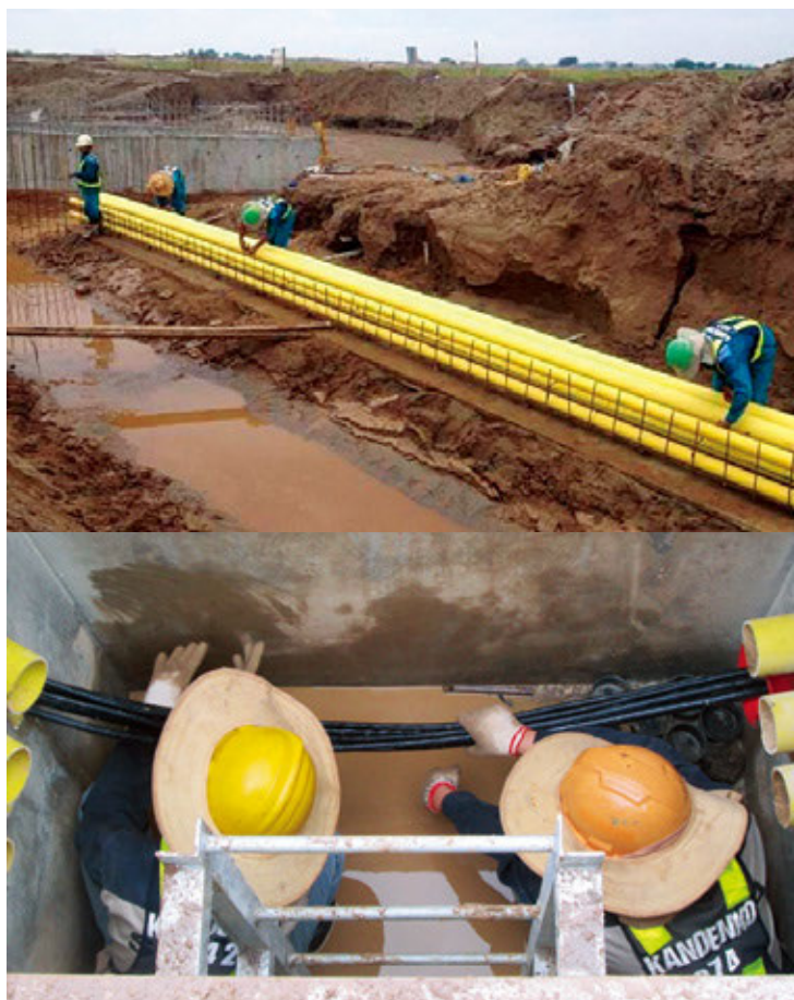
Pipe and cable laying operations were made complicated because of sludge.
