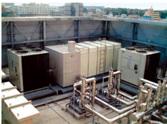
Ice-based thermal storage air conditioning system (Ibaraki Branch)
