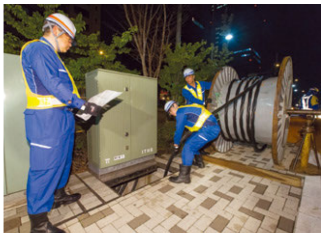
Laying cable for underground power distribution facilities
