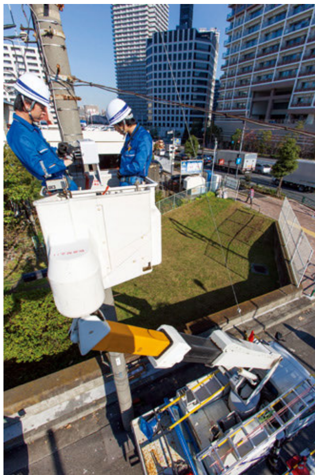
Installing a smart meter data aggregation device
