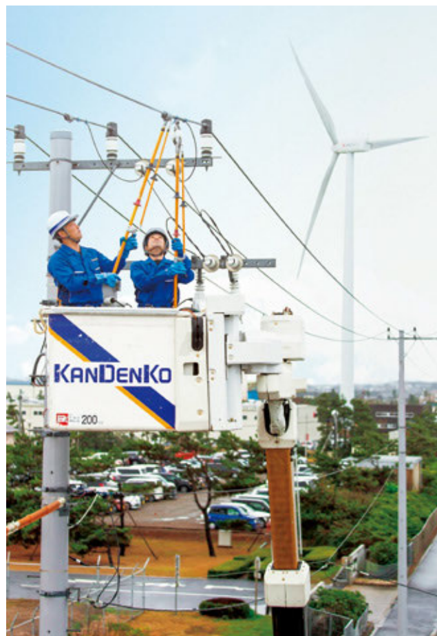
Work on overhead power distribution lines using hot sticks
