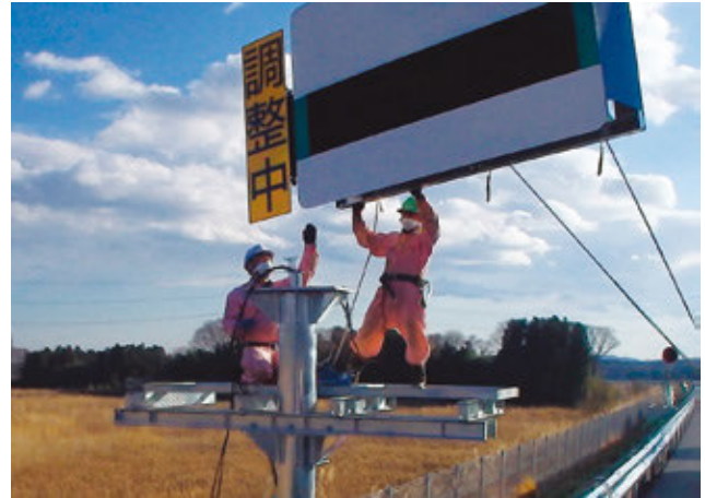
Installing an expressway information board
