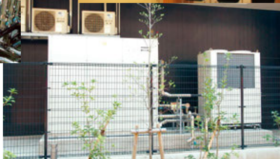
Kandenko's hot-water supply system for industrial use, "EcoCute Q" (Kawasaki Representative Office)
