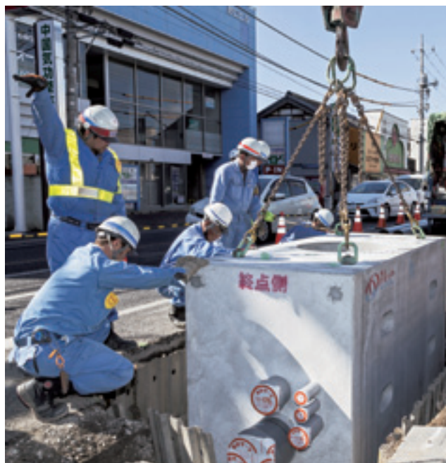
Installing a joint utility tunnel for electric power lines
