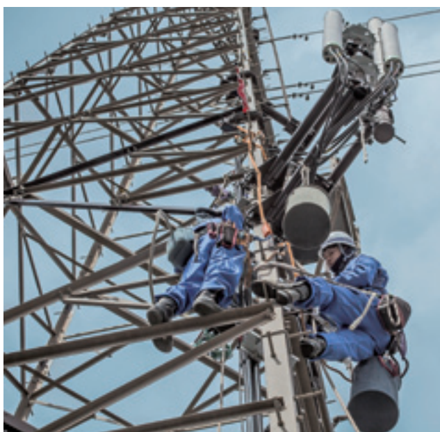
Installing a wireless telecommunications antenna
