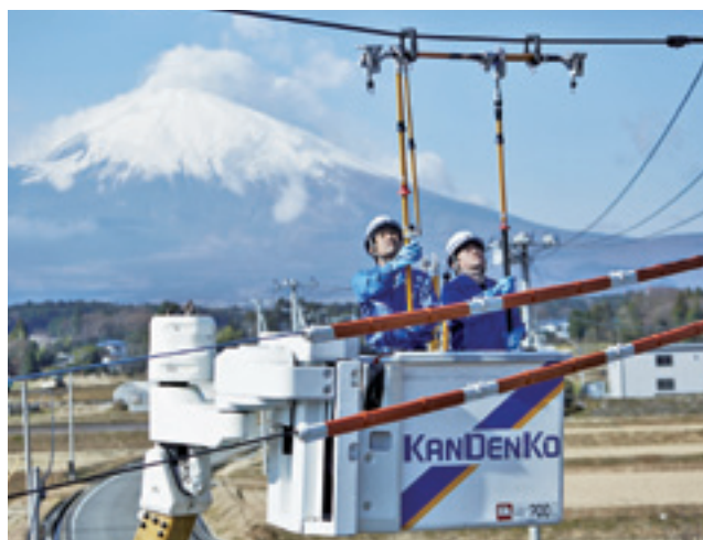
Work on overhead power distribution lines using indirect live-line techniques
