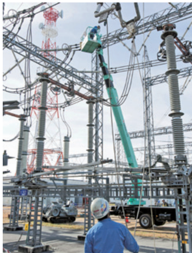
Stringing overhead power lines in the grounds of a substation
