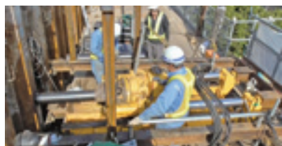
Anti-quake reinforcement work for railway tracks using small-bore tunnel drilling method
