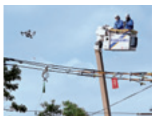
Drone used for work on overhead power distribution lines
