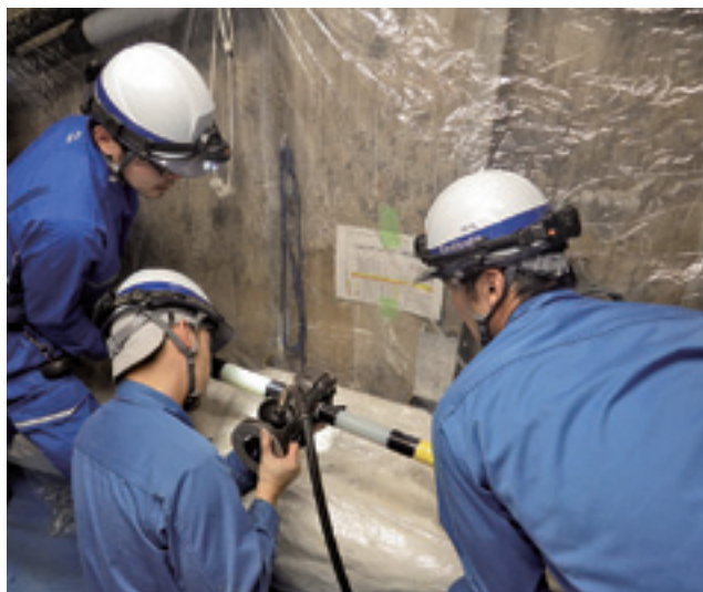
Connecting underground transmission cables
