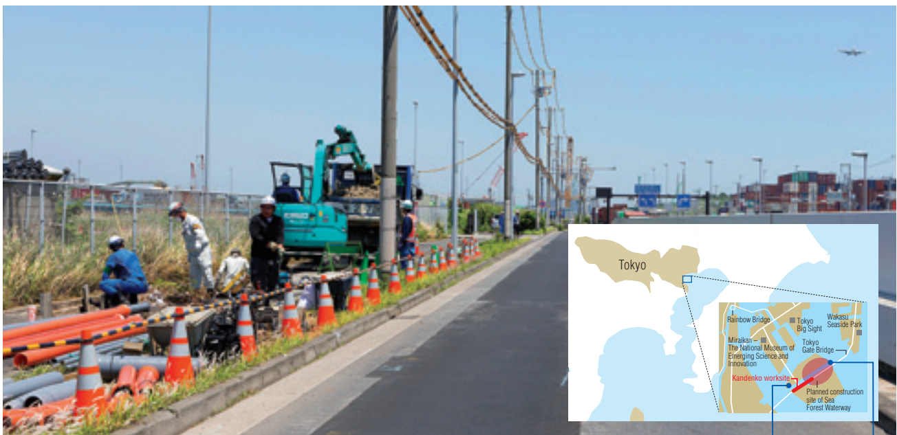
At this worksite, some 15 workers take part in night and day operations undergrounding power lines
