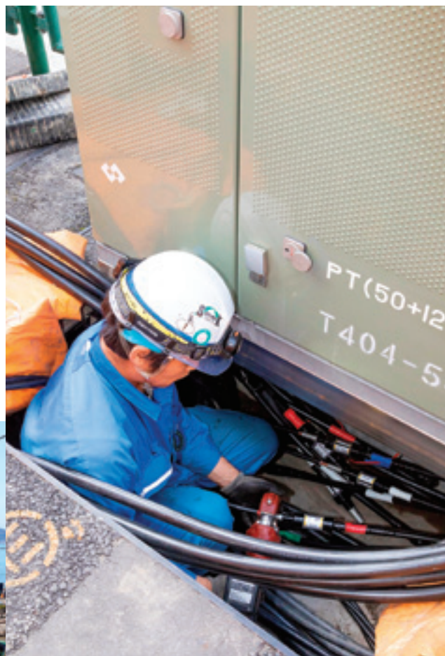
Connecting underground power distribution cables
