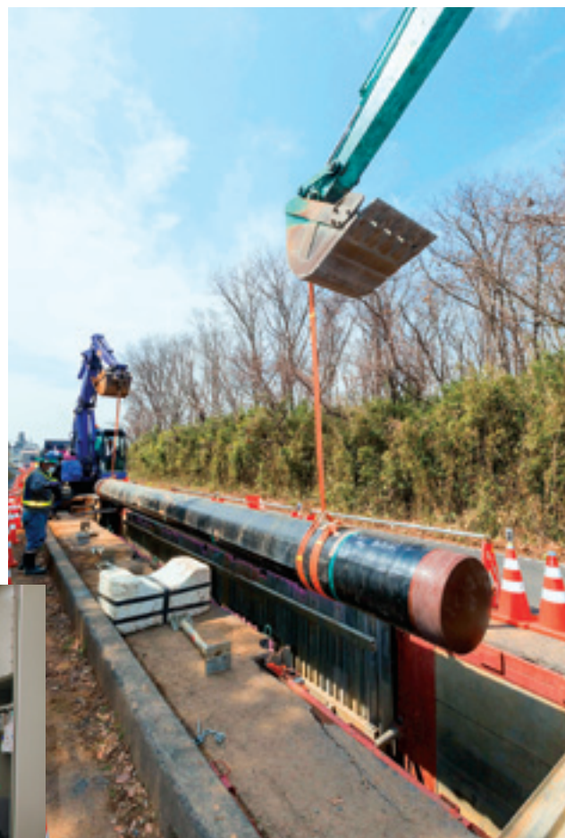
Laying an underground gas pipe
