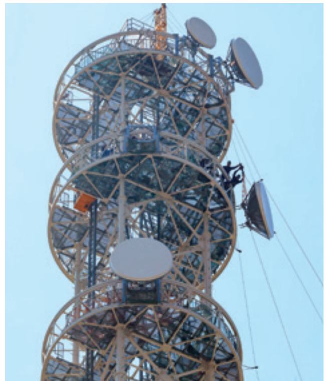
Installing a wireless telecommunications antenna
